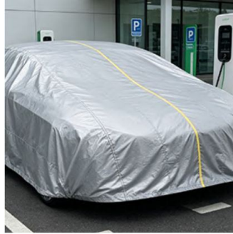
EV charging stations
